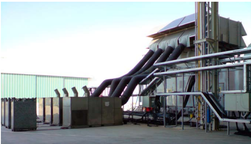
Pre-heating new power plant in Hungary.
