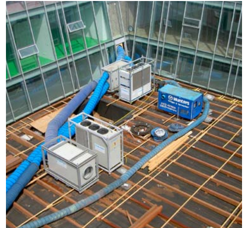
Temporary cooling of floors.
