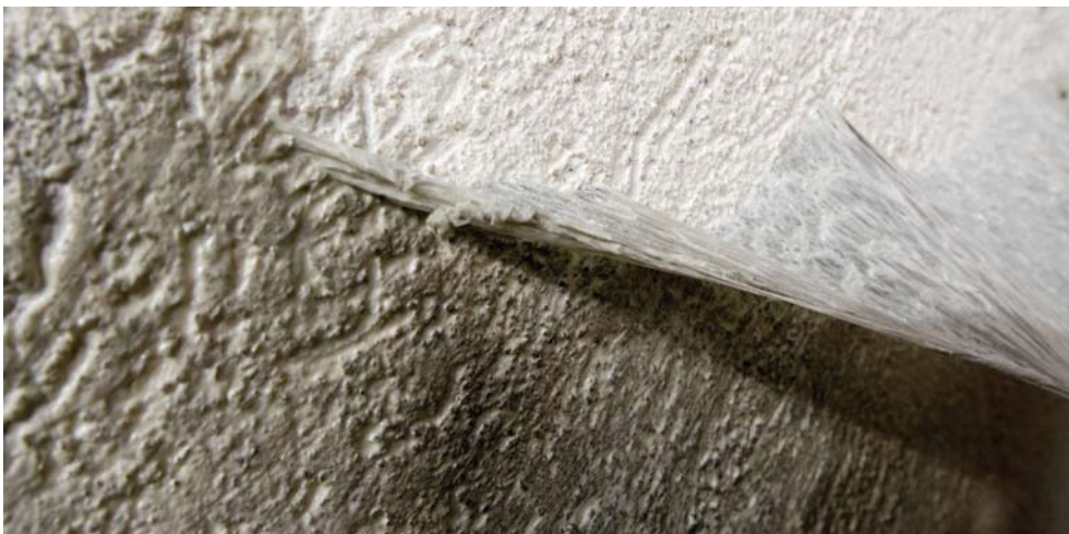
Removal of the transparent peelable skin once polymerisation is complete.
