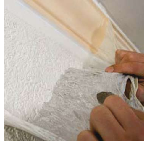
DeKonPeel® being removed as a peelable layer.
