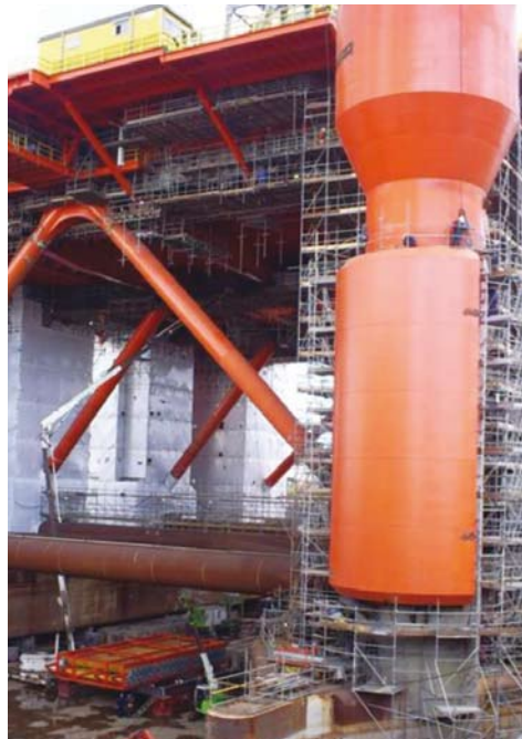
An oil rig being painted. The dehumidifiers protect the steel pillars from corrosion during blasting and before painting.
