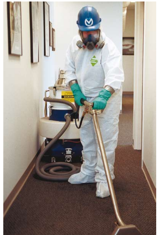
Water extraction equipment is used to remove moisture from carpet thus preventing the growth of mould.
