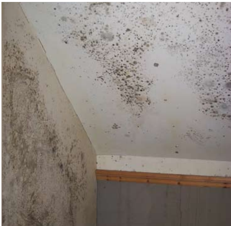
Internal mould growth.
