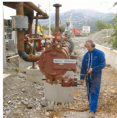
Monitoring pipeline dew point levels.
