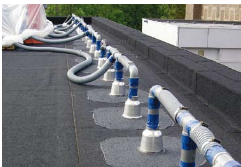
Drying equipment in place.
