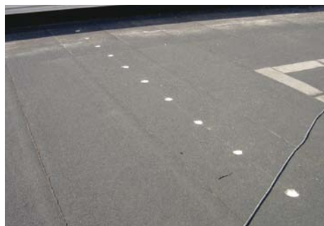
A fully restored dry roof.
