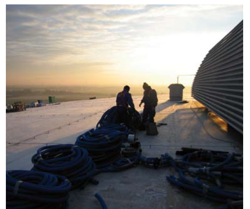
Rapid installation of equipment.
