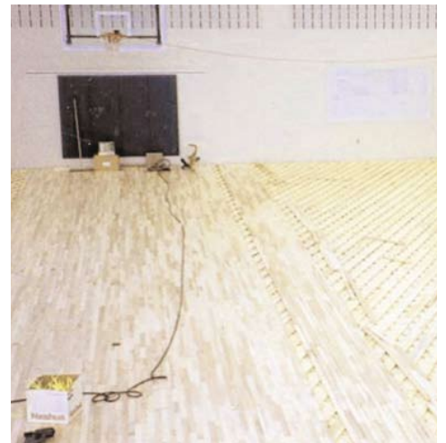
Restoration of wooden sports floor.
