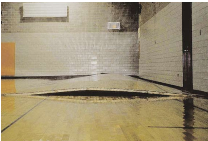
Lifting of sports floor.
