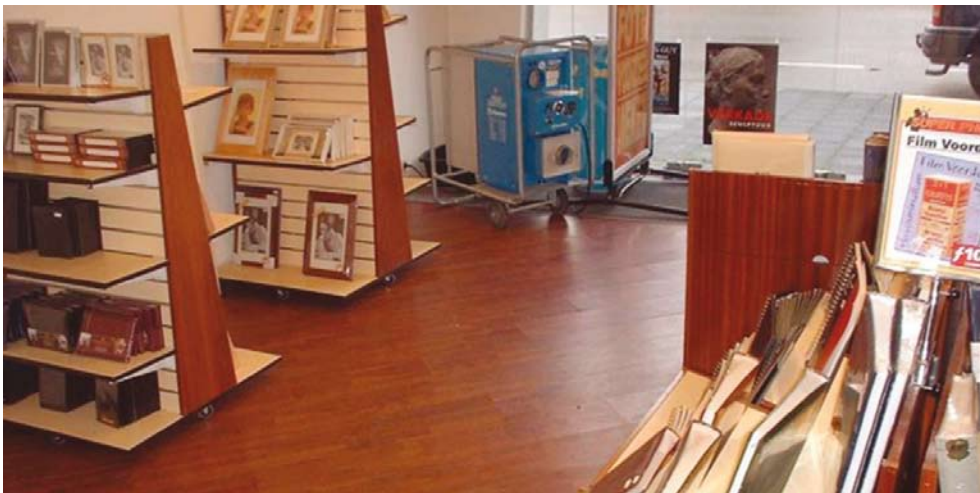
Dehumidification of damaged floor.
