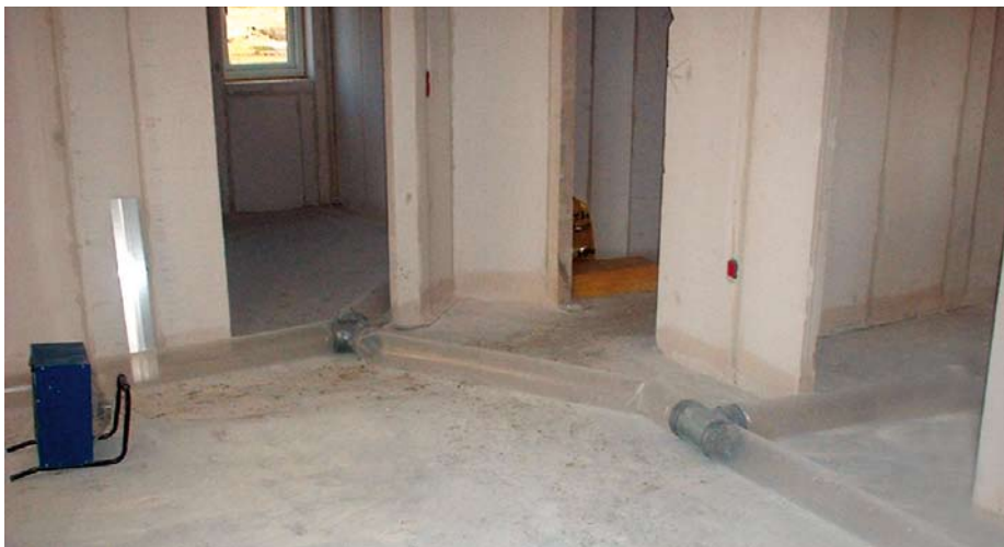
Hoses are used to evenly distribute the air.
