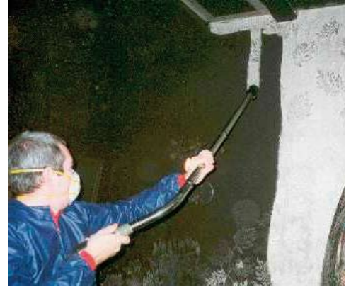
Vacuum extraction to remove loose carbon contaminants from building surfaces.
